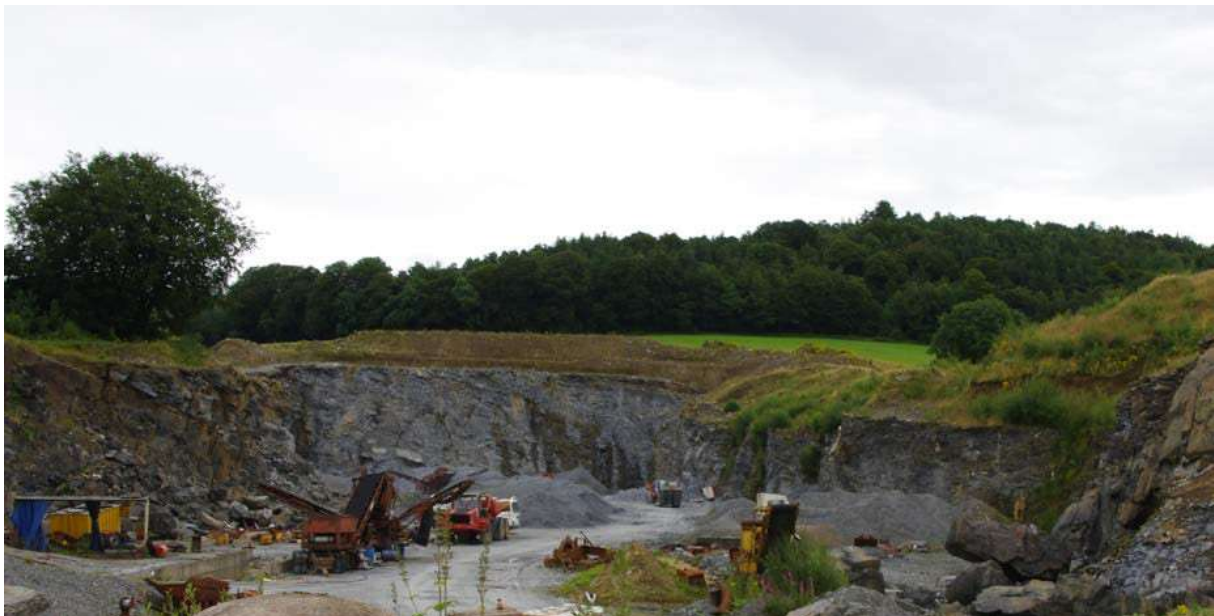
Plate 5. 1 Photo of the Quarry Working area (QWA) with crushing and screening plant
